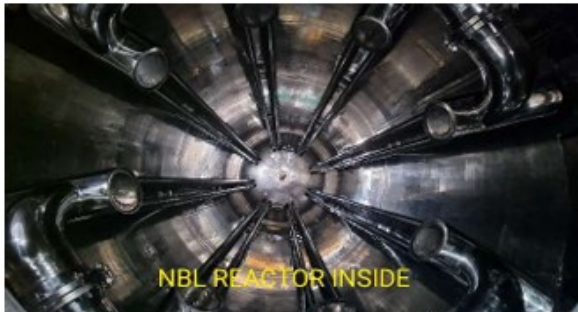
LG Malaysia NBL Reactor Internal
